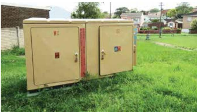
Figure 1: Mini-substation containing an 11 kV/400 V transformer, an 11 kV ring main unit and LV circuit fuses.
