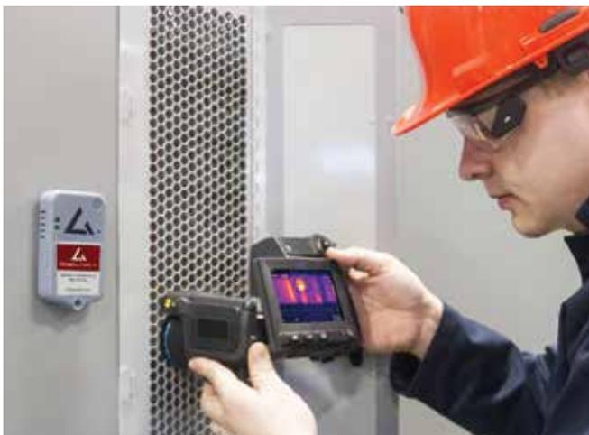
World leaders in switchgear manufacture have tested the IRIS Polymer version of the IR window and now offer Polymer IR windows as options when manufacturing switchgear.
